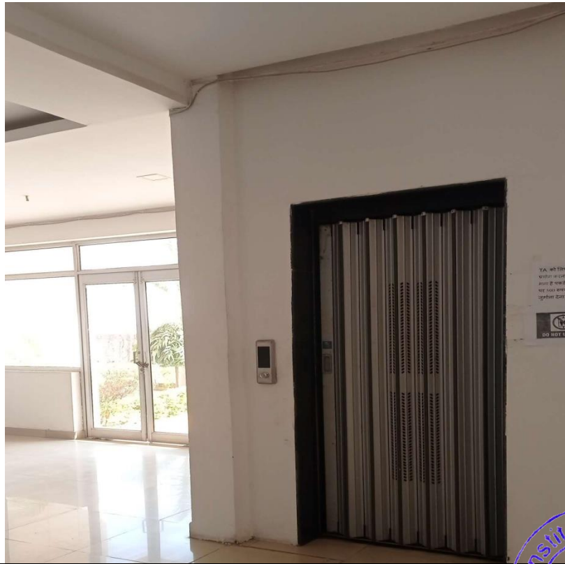
Lift in Library Building
