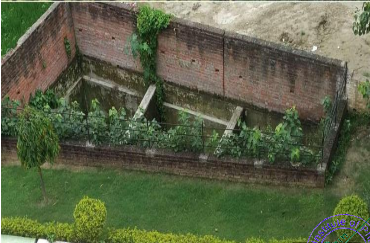
RAIN WATER HARVESTING
